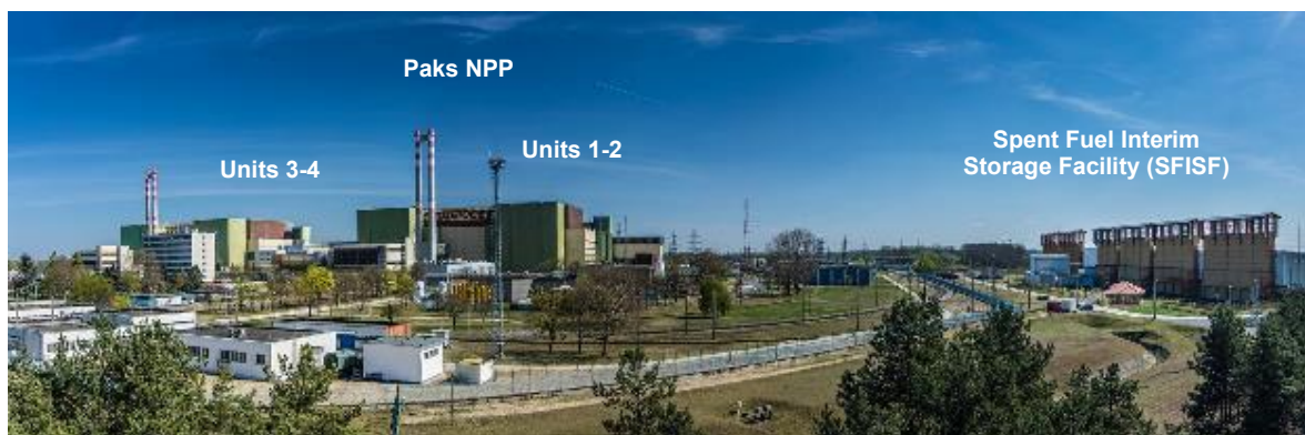
Figure 2.2-1. The SFISF and the main buildings of the Paks NPP
