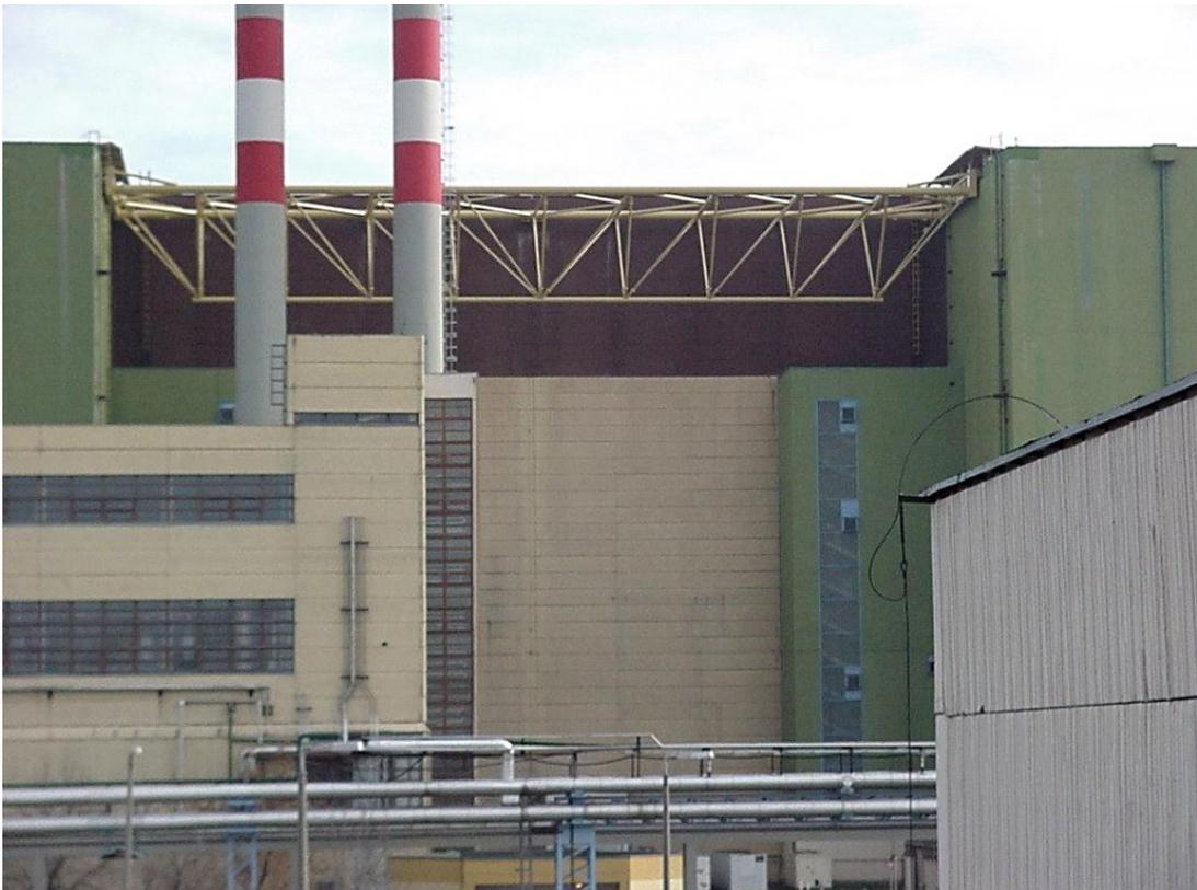
Figure 3: Bridge structure between the bubble towers for reinforcing the reactor building structures
