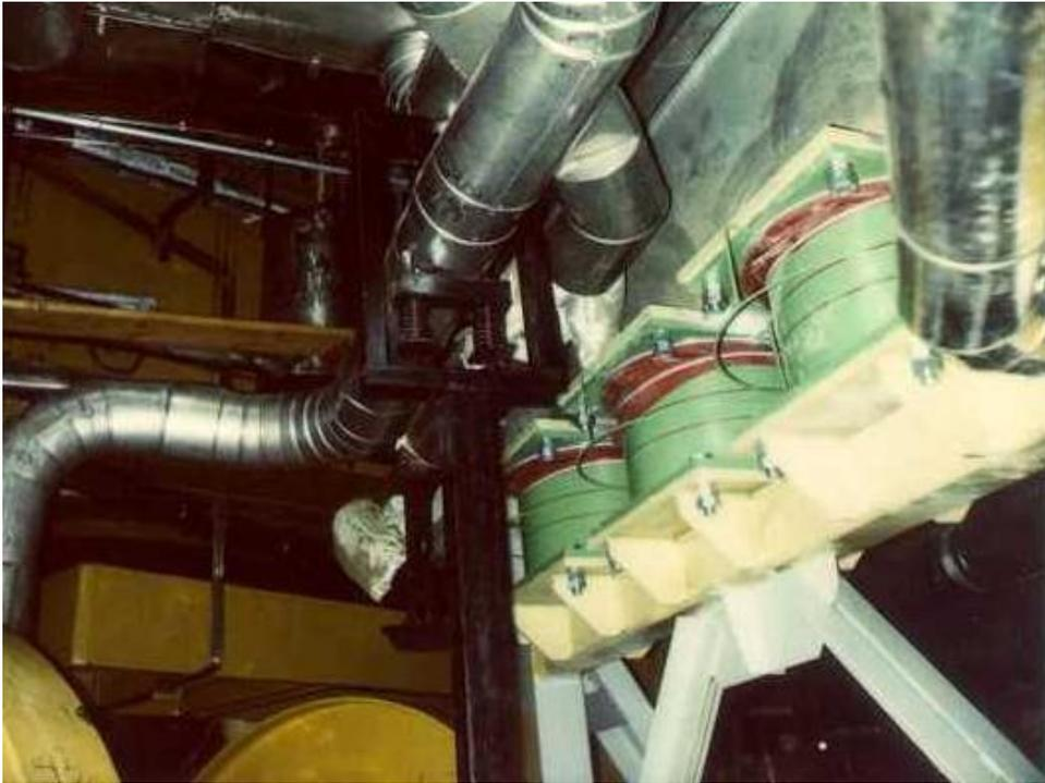
Figure 1: Viscous vibration dampers beneath the steam generators
