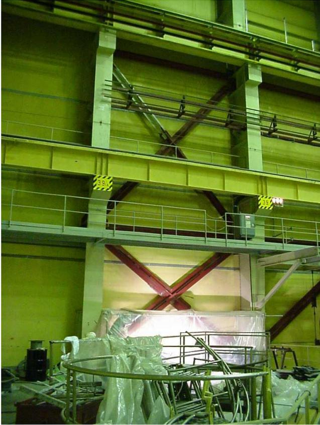
Figure 2: Longitudinal reinforcements in the reactor hall
