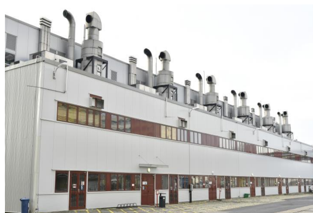
The diesel generator building for Units 1-2
