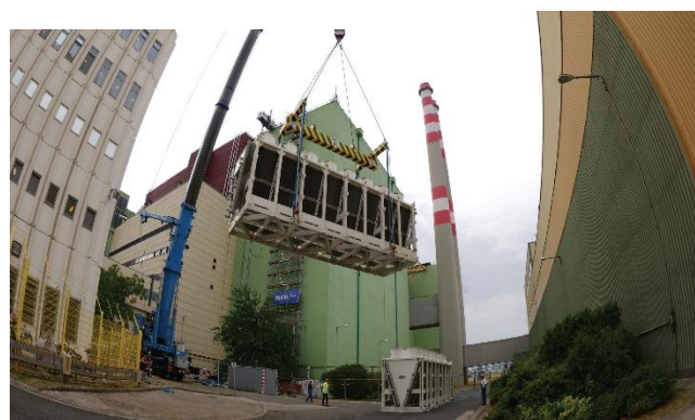
Installing an air cooler on top of the localisation tower
